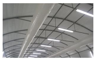
MC285, characterized by the high UV resistance, the white inner cover 7SE, characterized by its flame retardancy and for both their tensile strength and wear-resistance. These covers also hardly show any signs of shrinking or stretching at large temperature differences and are used in many climates. Even in areas with a great deal of wind they provide the grower a long-time guarantee for problem-free accommodation for his mushrooms.
