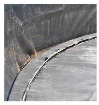
The floating cover is installed on top of the liner, after installation is finished, the manure/effluent is pumped between the liner and the floating cover. Floats with outlets under the cover keep the membrane floating, even after heavy rain fall. As a cover, high UV resistance of the TenCate Nicolon® C119/800 membrane is one of the most important properties.
